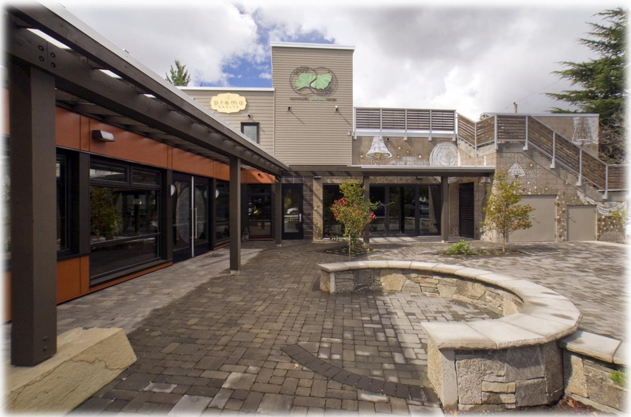
Above: Exterior courtyard featuring permeable pavers & benches made with re-used concrete spoils
