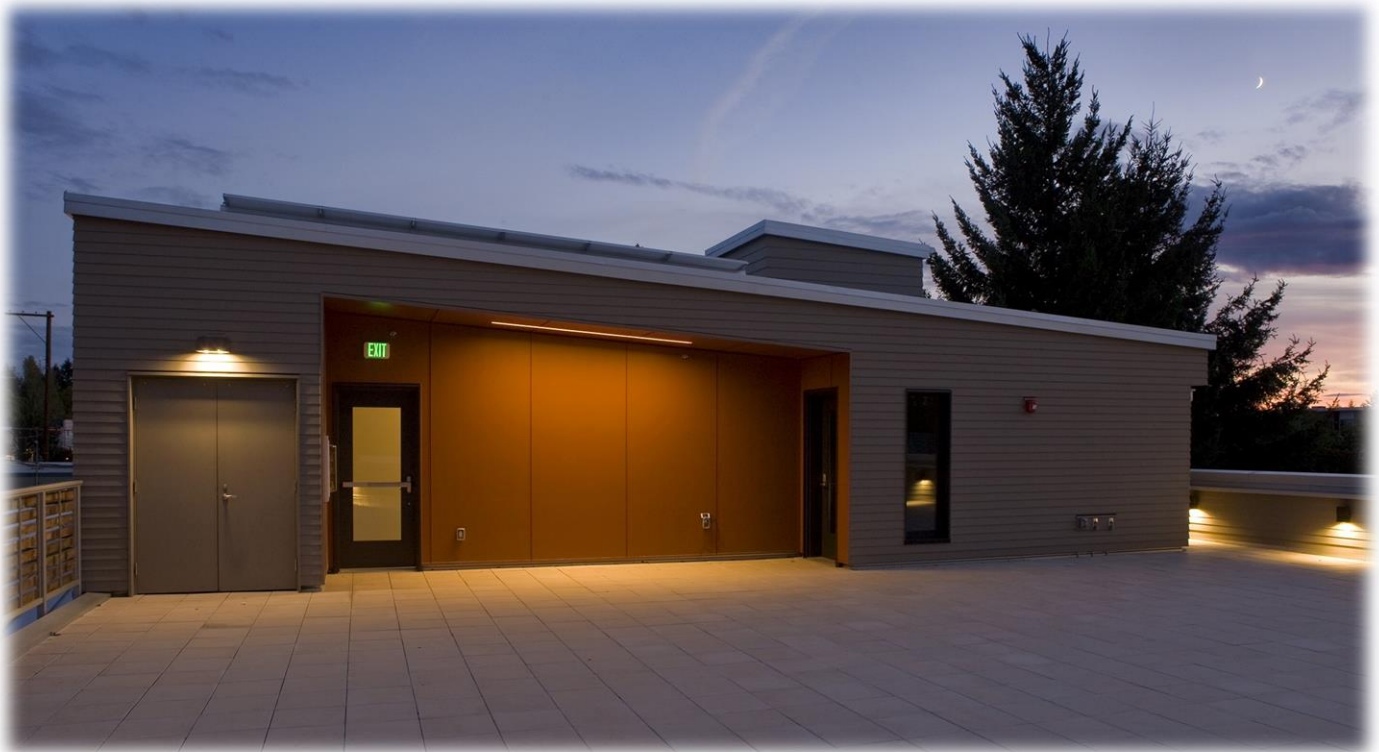
Above: The rooftop terrace includes an ADA unisex bathroom and is served by the elevator
