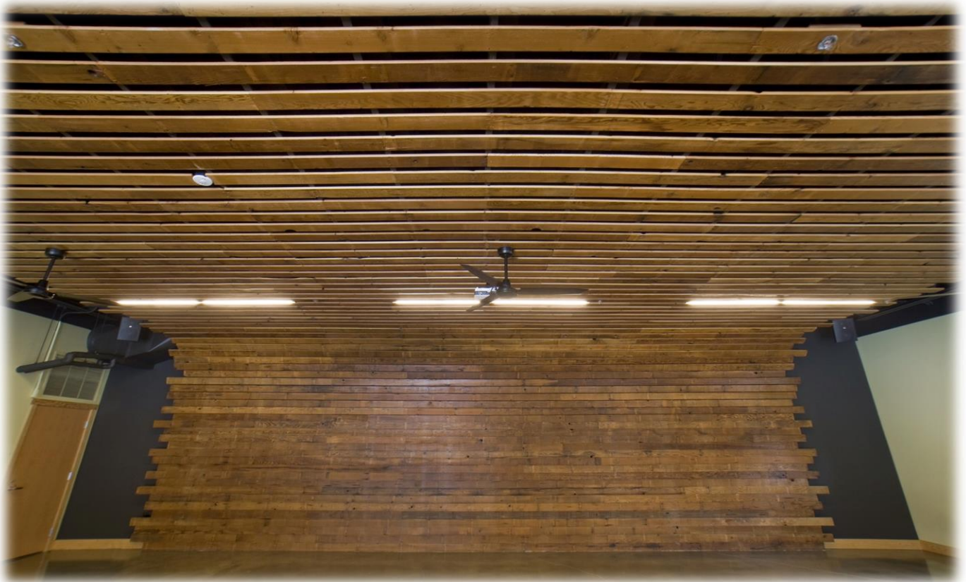
Above: Main studio wood wall and ceiling made from lumber re-used from the former buildings
